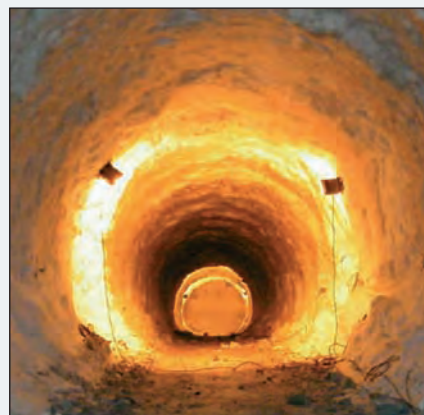
Figure 26 and 27 - 5m diameter frozen pilot tunnel before and during breakthrough of the 10.6 m diameter TBM.
