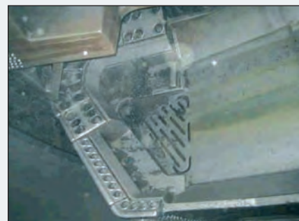
Figure 9 - Dewatering grids along muck channel.
