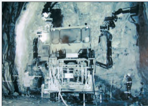
Figures 4 and 5 - The first two attempts: open gripper TBM and drill & blast methods
