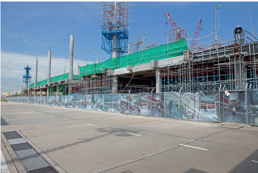
Climbing formwork at the foot of the runway in Phnom Penh.
