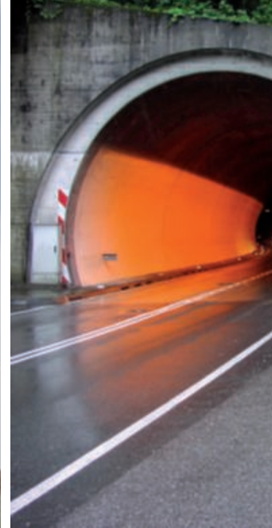
BREGENZ TUNNEL IN AUSTRIA
