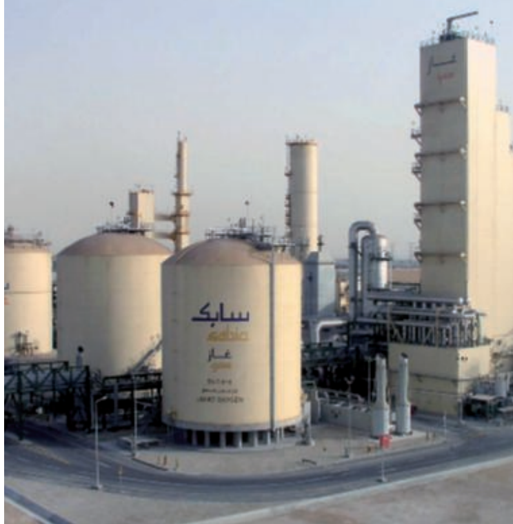
OXYGEN PRODUCTION FACILITY IN SAUDI ARABIA
